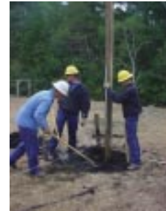
CCEC linemen make final adjustments before setting the poles.
